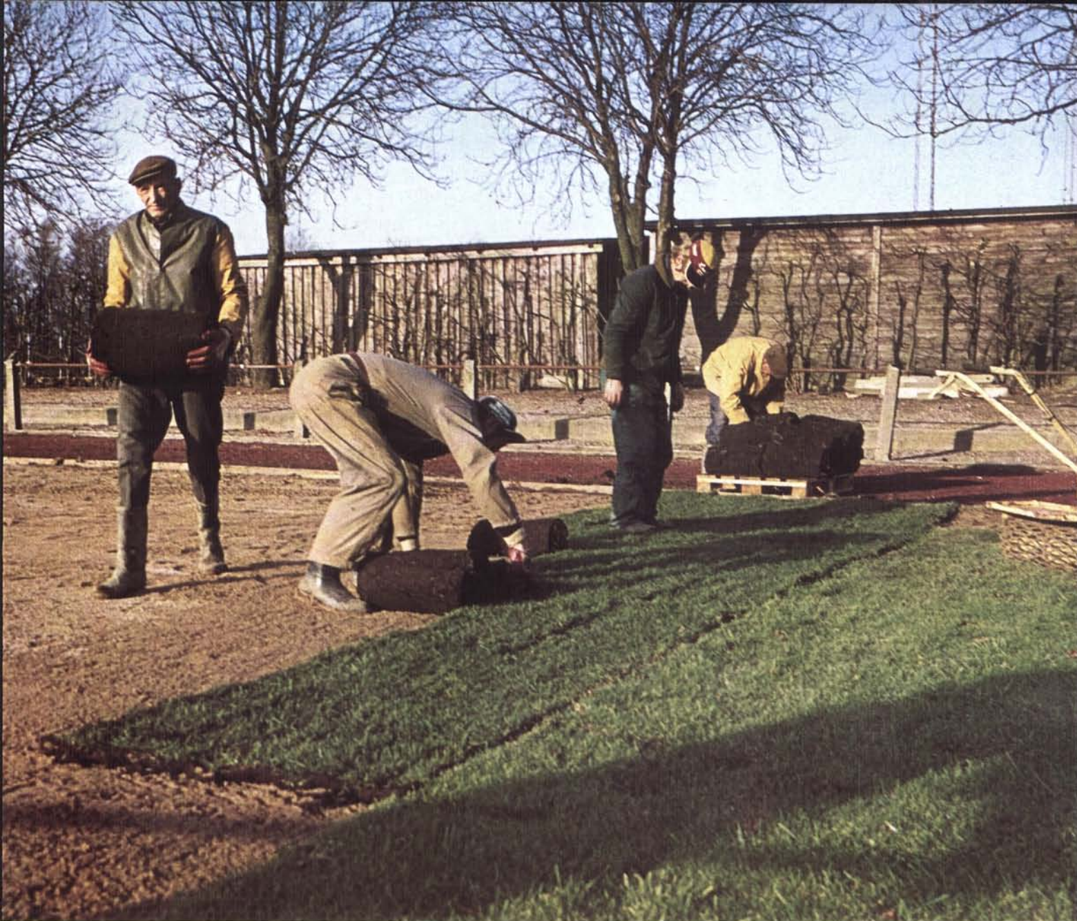
Laying prefabricated GREENLUX lawn turf.
