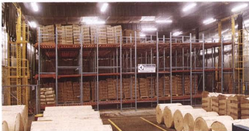
A. Interior picture of the finished goods store of the garbage bag factory, showing also the roller boxes and the arrangement for automatic stocking (see sketch outline on page 18).
