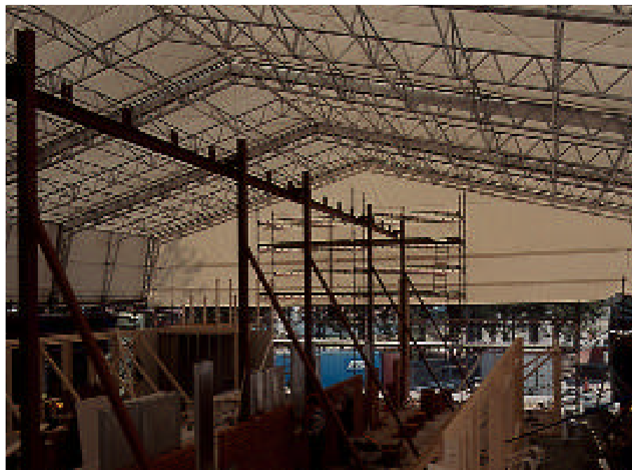
With Jonsered's system for "dry building" sites, construction work can take place indoors! Among other things, this can help to prevent future mold problems.
