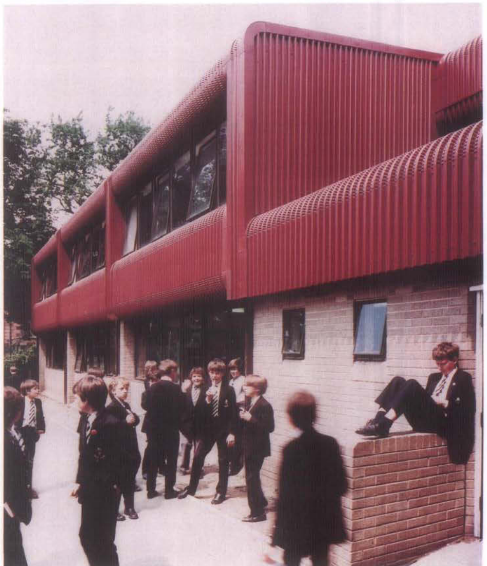
Gränges Aluminium is highly successful in the British market. The picture shows Korrugal structural sheet for roof and cladding at a school in Liverpool.
