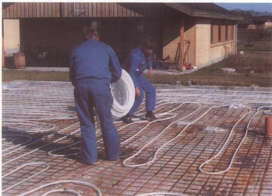
Wirso's under-floor heating system saves 15 percent of the energy compared with conventional radiators. It is suitable for installation in apartment blocks, public premises, sports halls, stores, etc.
