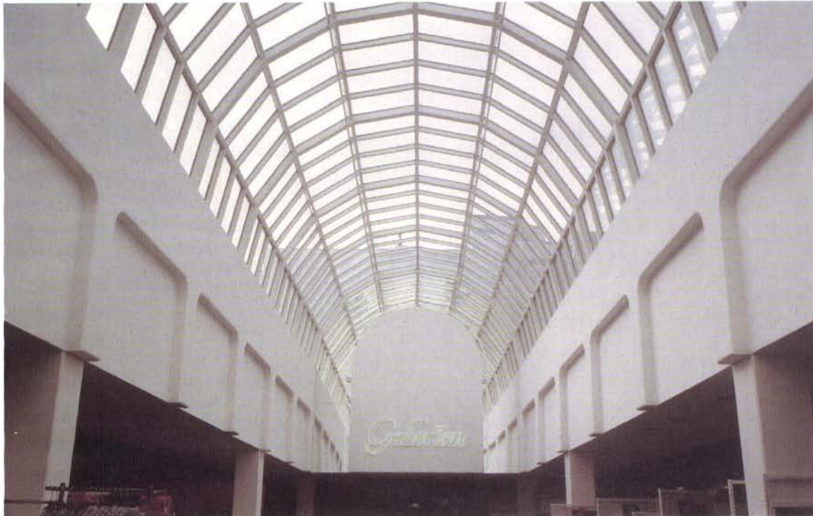
The building industry is Gränges Aluminium's largest customer. Here SAPA's aluminium profiles are used to cover a newly-built shopping centre in Malmö.
