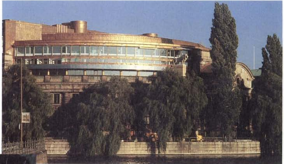
The converted Parliament Building in Stockholm has been roofed with copper cladding.
