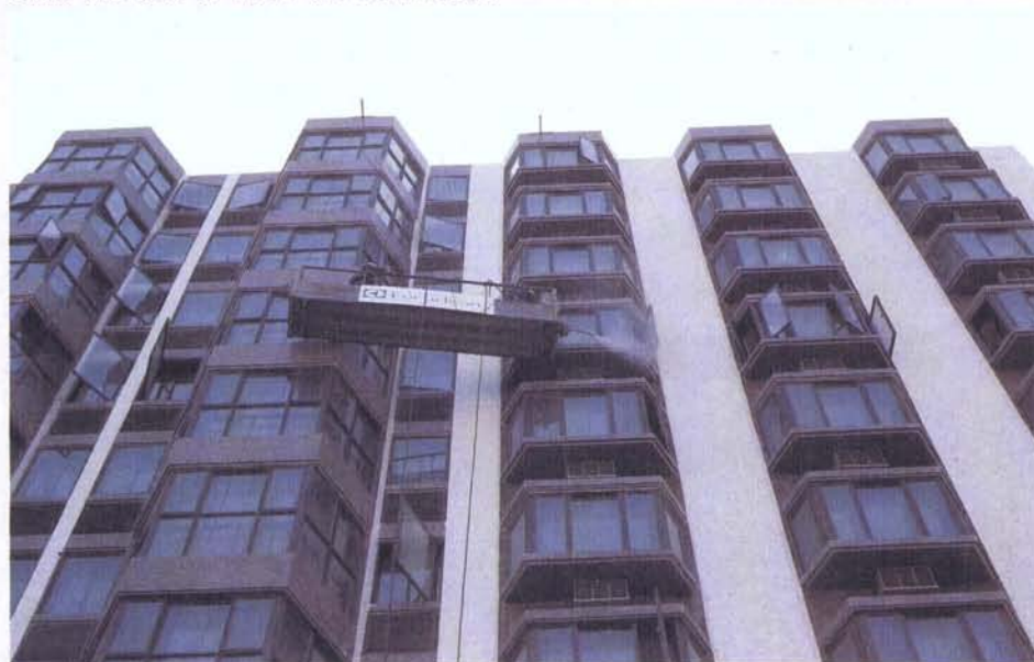
Cleaning building facades in Hong Kong.
